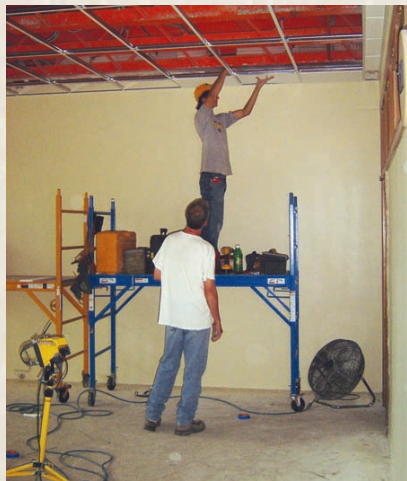
Workers install the new ceiling in Classroom C
